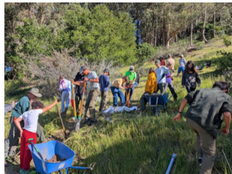
Scouts busy at work installing the bat house pole and sign post
